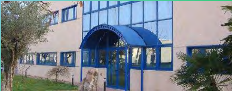
Hiref factory in Padova: offices & sanitary water: 18 kW
