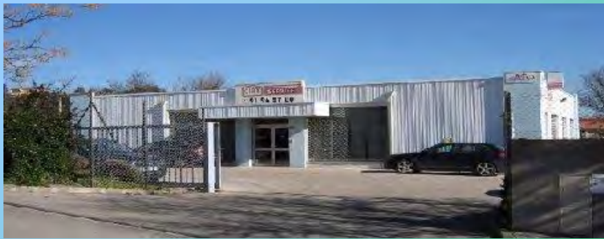
Ciat subsidiary offices in Septemes les Vallons: 30 kW
