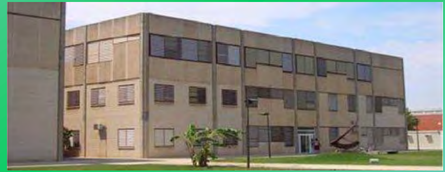
University of Valencia campus offices building: 18 kW
