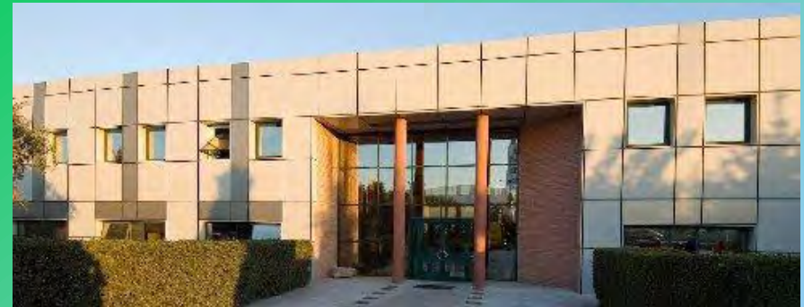
Edrasis headquarters office building, Athens: 55 kW
