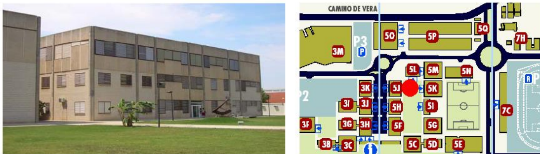
Figure 1.- 5J UPV Building view and location.
