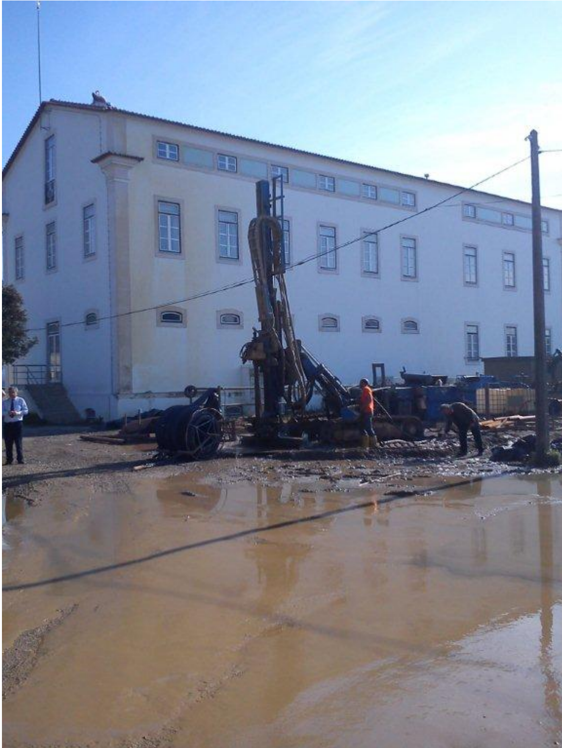
Visiting the Coimbra demo site: BHE construction works
